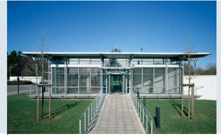
Reception building, Lüdenscheid
